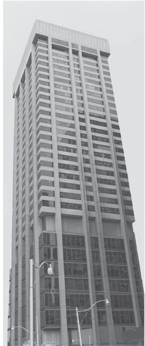
Columns in a high-rise building.
