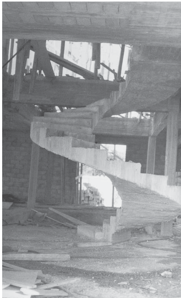
Reinforced concrete helical staircase.
