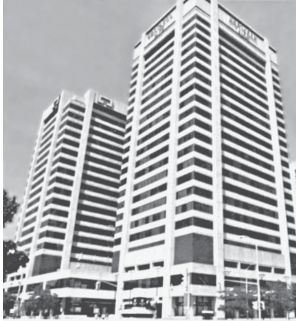
90° V-shape beams, London, Ontario, Canada.
