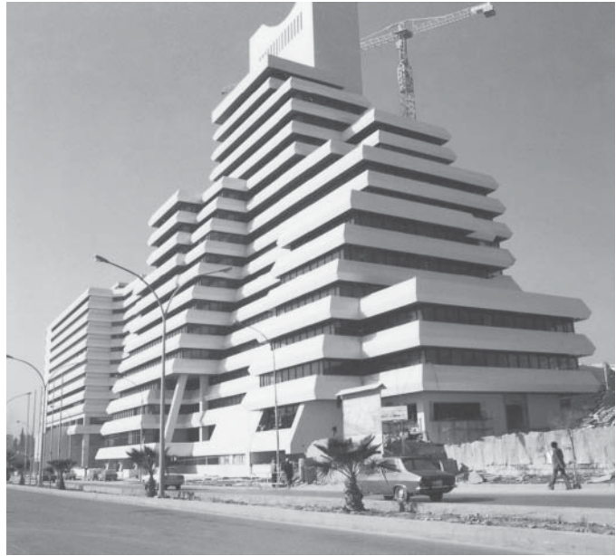
Reinforced concrete office building, Amman, Jordan.
