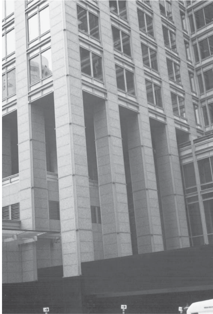
Long columns in an office building.
