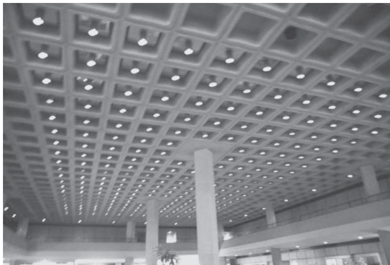
Waffle slab with light fixtures at the centers of the squares.
