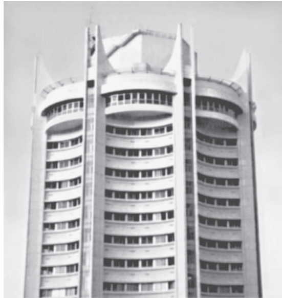
Circular beams in an office building.
