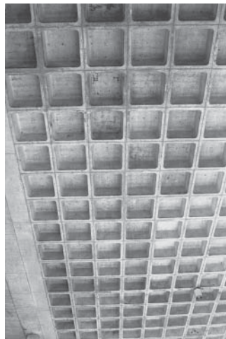
Waffle slab (looking upward).
