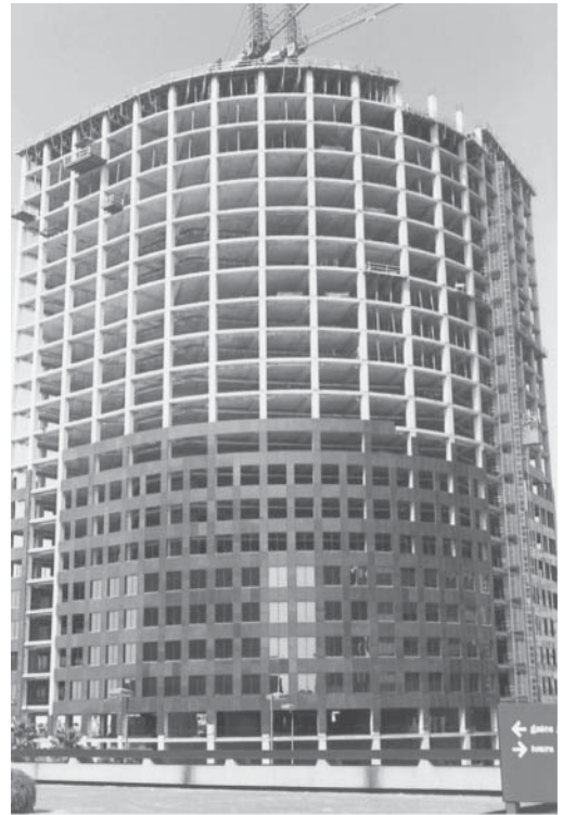
Office building under construction, New Orleans, Louisiana.
