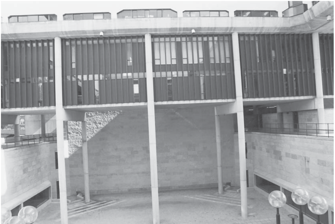
Columns, University of Wisconsin, Madison, Wisconsin.
