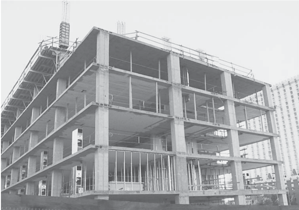
Flat-plate floor system.
