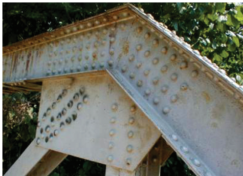
Fig. 29.6. Chain riveted joint.
